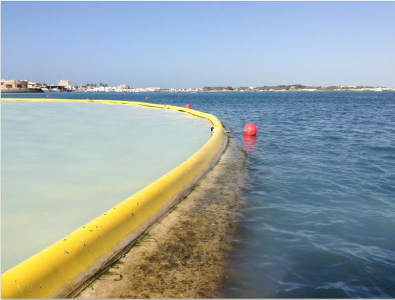
In terms of particle size, sand is classified as size between 0.05mm-2.0mm, silt between 0.002mm-0.05mm, and clay less than 0.002mm. By basing silt curtain material selection only on permeability assumptions defined by ASTM D4751, incorrect conclusions can be drawn that these particles will pass through the fabrics and as a result lead to incorrect selection of fabrics to
