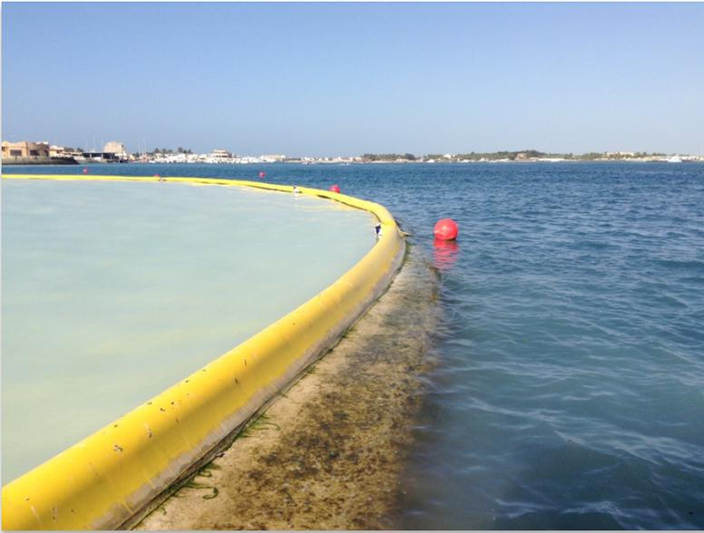
The aim of a silt curtain is to act as a settlement pond and allow the silts time to settle within the contained area to reduce the spread. Silt curtains are not designed to impound water completely, and it is reasonably expected that some silts will move underneath. By allowing the silts to settle from the upper portion of the water body, the area of spread will be limited significantly, and the chance of the silts being re-suspended will be reduced.
