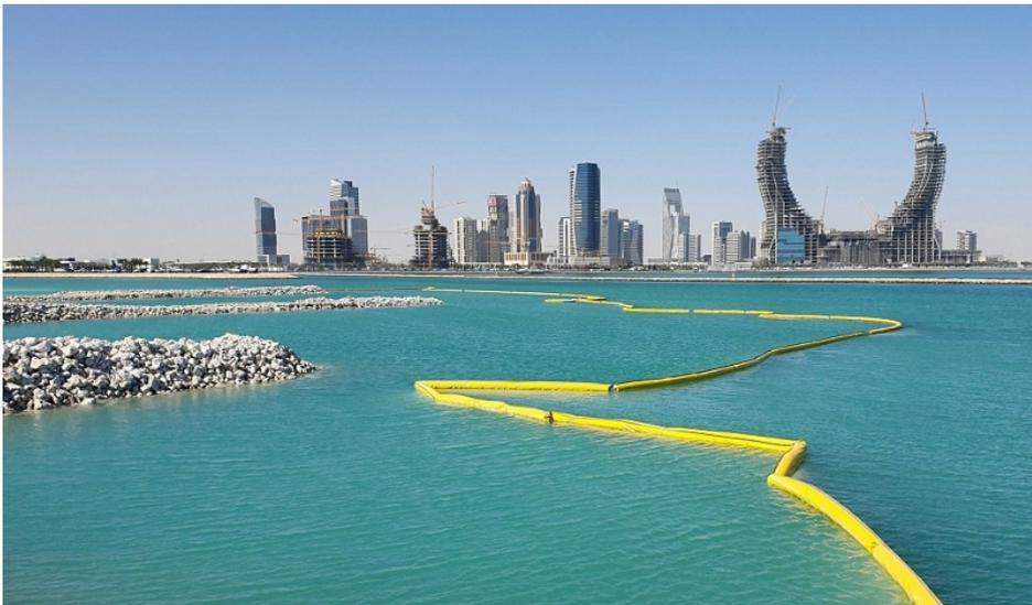
*Ecobarrier silt curtain type III in use © Ecocoast*
