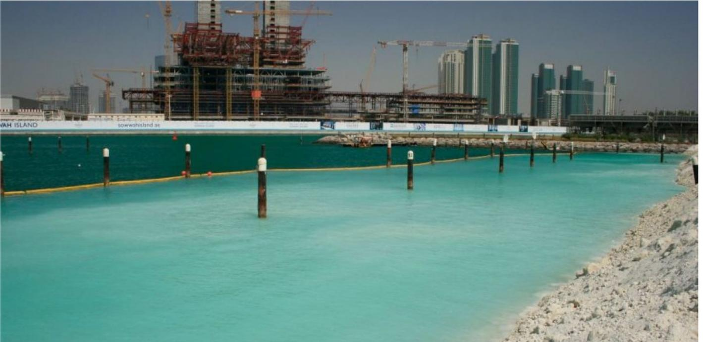
The silt curtain barrier provides a clearly visible line, showing the dramatic difference in turbidity. Photo: Ecocoast 07 Dec 2020
